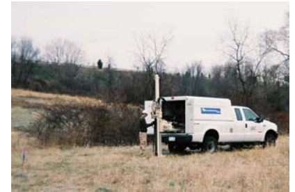
Direct Push Soil Borings
