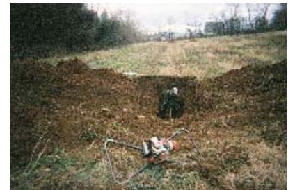
At Depth Infiltration Rate testing
