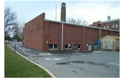
Photograph of groundwater treatment system area.
